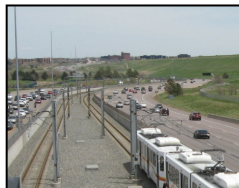
Figure 3.6 Fence Along LRT
