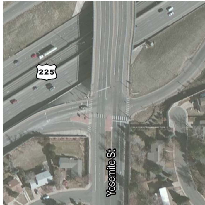
Figure 7. Northbound I-225/Yosemite Street Ramp Terminal
