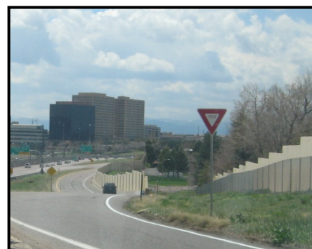
Figure 3.8 Sound Walls Along Southbound C-D Road
