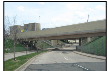
Figure 3.11 Southbound I-225 over Quebec
