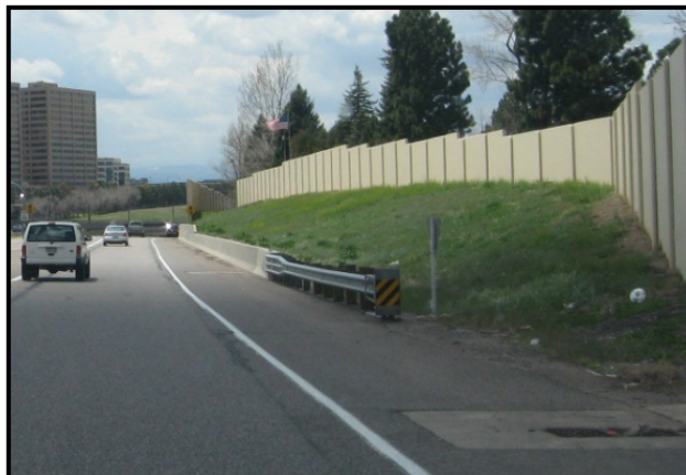
Figure 3.5 Guardrail Along Southbound C-D Road
